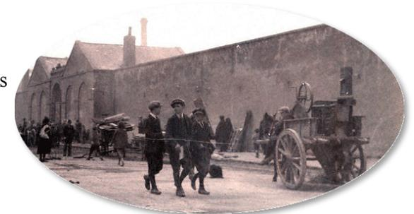
The former magazine store is listed on the record of protected structures for Limerick City and is noted as being of National Importance and 'an important and rare typology in Ireland'. It is a brick barrel vaulted single storey structure with limestone external finish and buttresses. This architecturally significant building has been restored while the new courthouse respectfully strengthens its presence.
